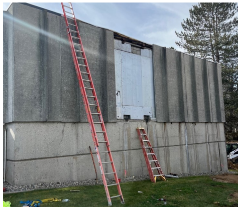
TE wall removal
